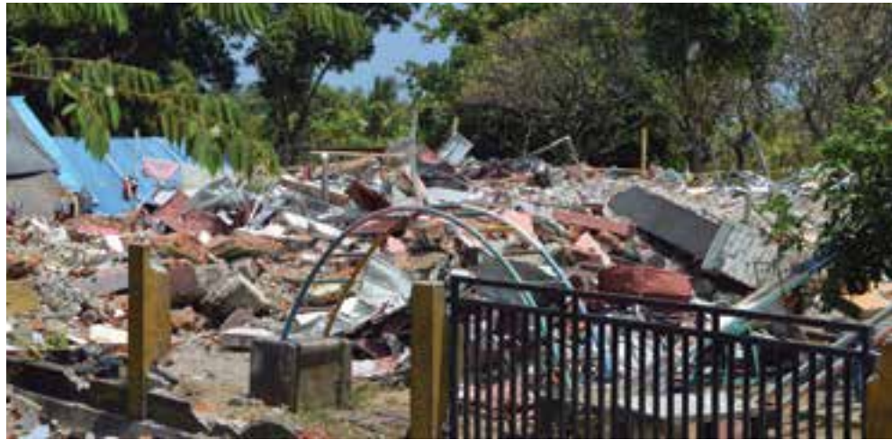
Above: the site of the village's kindergarten just after a devastating earthquake flattened virtually everything in the summer of 2018.
