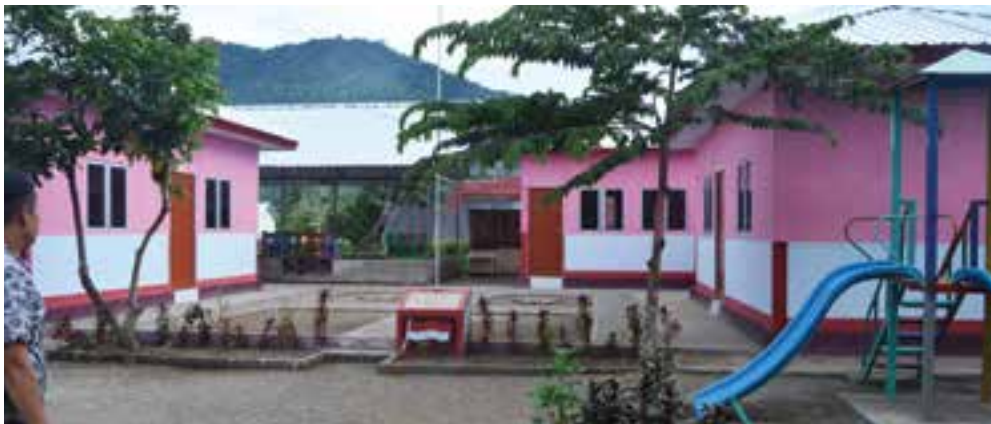
Below: the newly rebuilt and improved kindergarten buildings, including boys and girls washrooms, sinks and a playground.
